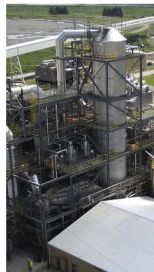
Fig. 15. Schematic of the chilled ammonia process for CO 2 capture (left) and the 20 MW pilot plant at the AEP Mountaineer station in West Virginia (right); Photo courtesy of AEP.
