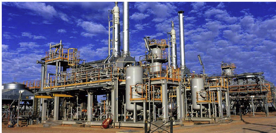
Fig. 13. An amine-based CO 2 capture systems used to purify natural gas at BP's In Salah plant in Algeria; Photo courtesy of IEA Greenhouse Gas Programme.
