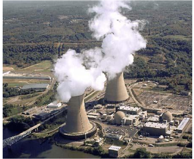
Nuclear plant near Shippingport, PA Source: www.nrc.gov
