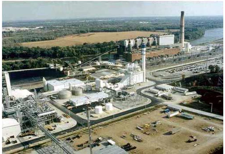
An Coal-to-gas Plant in Indiana
