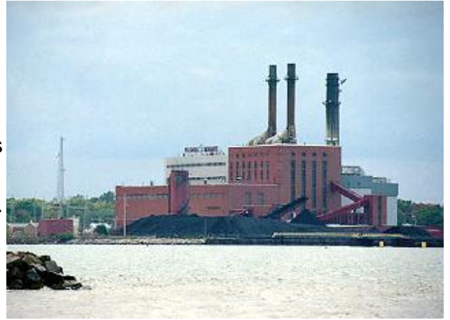
Biomass-coal power plant in Dunkirk, NY Source: www.ens-newswire.com
