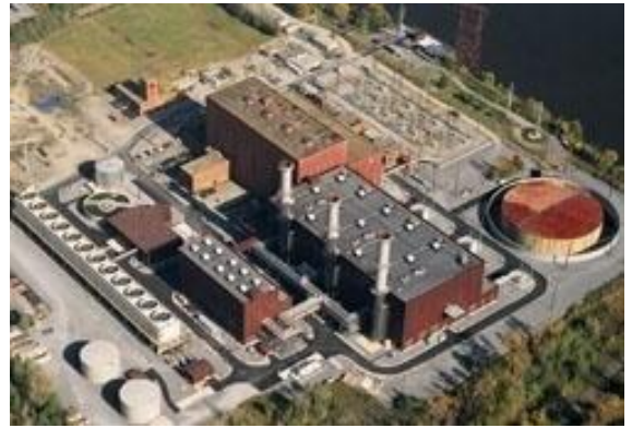
Natural gas plant near Albany, New York. Source: www.pseg.com
