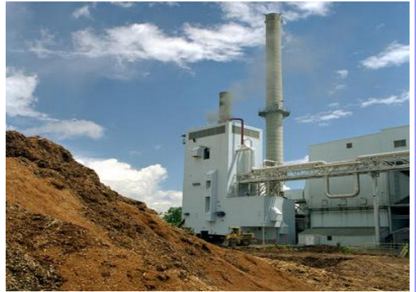
Biomass power plant in Burlington, VT, Source: www.nrel.gov/biomass/photos.html
