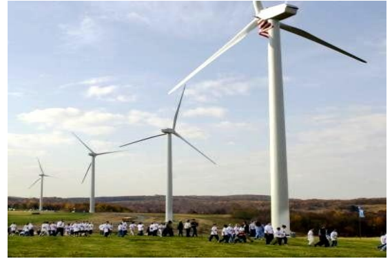
Modern wind turbines in Somerset, PA Source: www.solutions-site.org/
